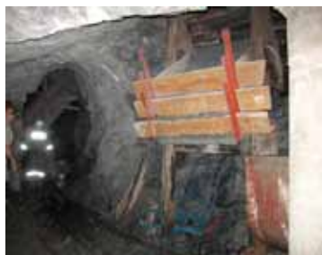
Newly installed ore pass
