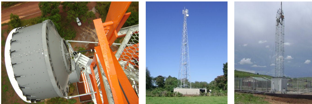
NSS-built GSM lattice masts, South Sudan
