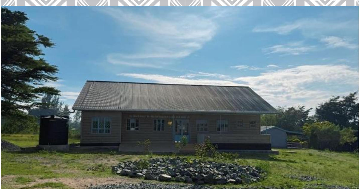
The newly constructed Kibisem Health Center
