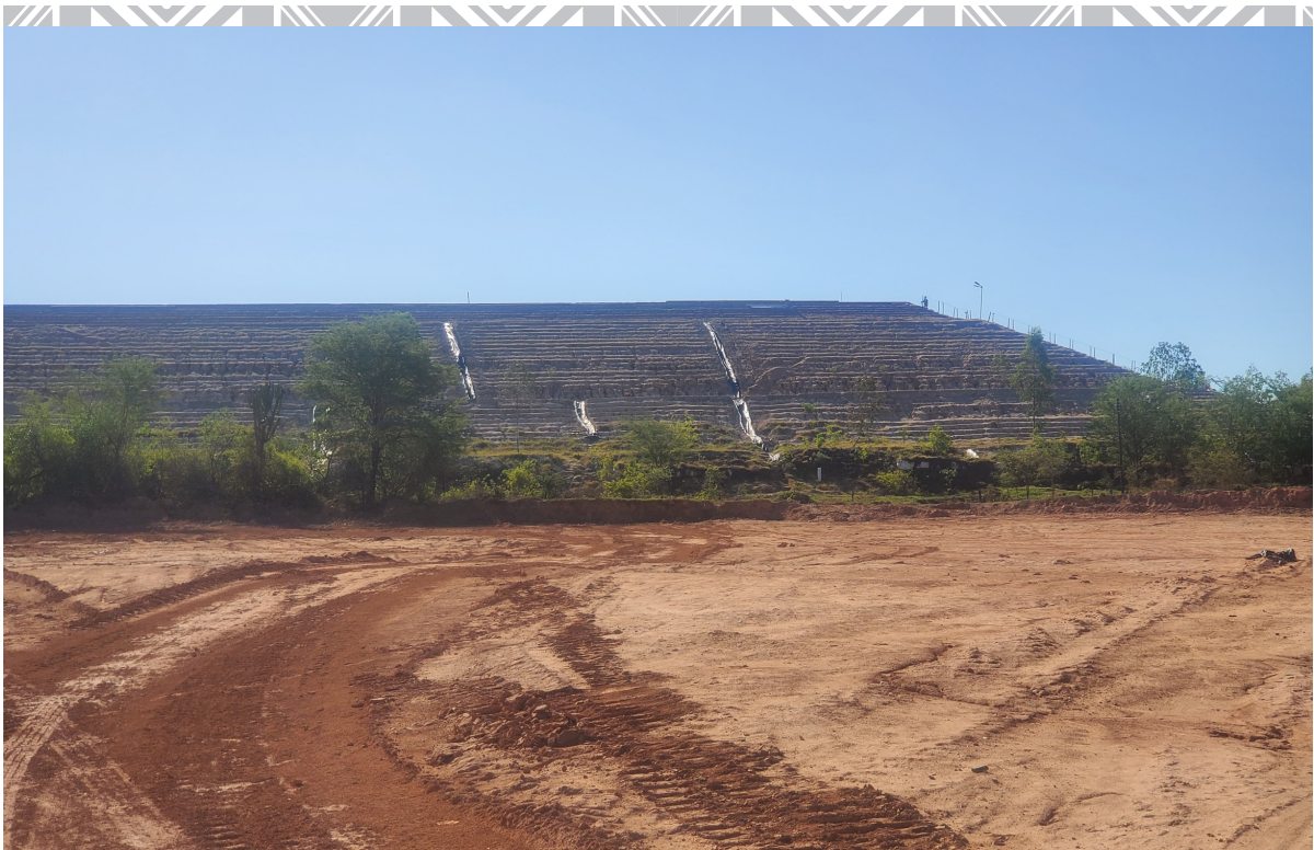
A section of one of the tailings dam in Venice Mine Complex
