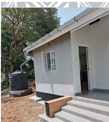
Newly renovated principal's house
