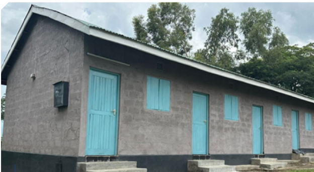
One of the teachers' accommodation blocks constructed by KGML in May 2023
