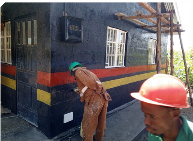
Renovation of Chepswerta Police Station by Karebe Gold Mining Ltd
