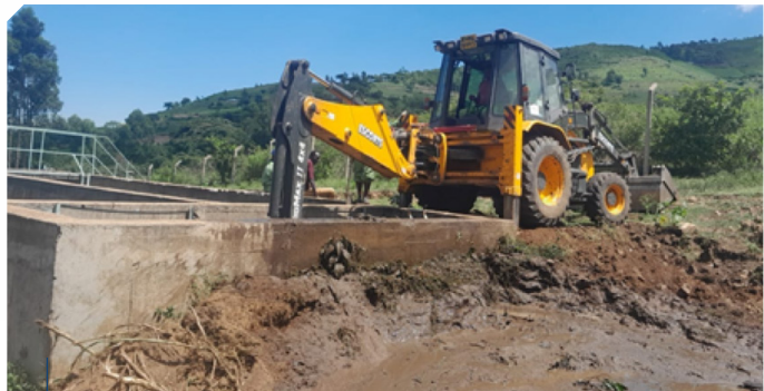
Cleaning one of the community’s water intake points maintained by Karebe after heavy rains in May to clear mud from the water.
