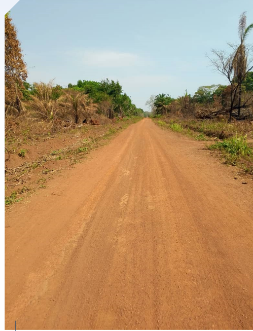
A section of the newly constructed 15km Nzara - Mborizanga road
