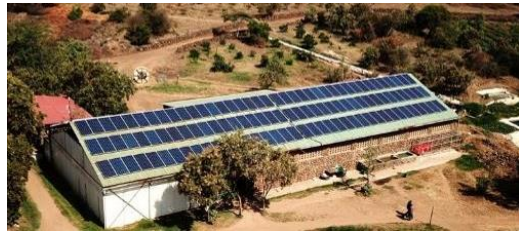
EQUATOR ENERGY INSTALLATION
