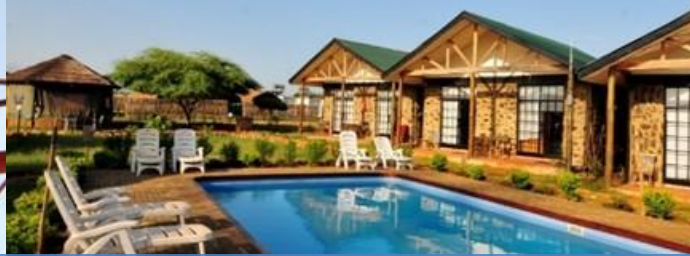
Maris builds No1 corporate serviced accommodation compound in South Sudan
